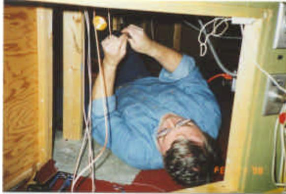
Selecting the wire was easy!! There is simply nothing better than the various LGB twin-lead wire products. It's color coded, easy to work with, and has more than enough current capacity. Did I mention that it's easy to work with! You don't have to fight with LGB wire. We used the black and white 50140 for all AC wiring. The 50130 orange and white wire was used for all control and EPL wiring, and the blue and red 51230 wire was used for DC track power.
